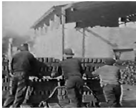
Workers moving bricks
