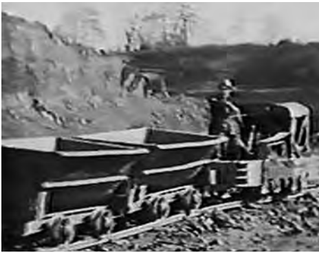
Rail Carts going to get filled
